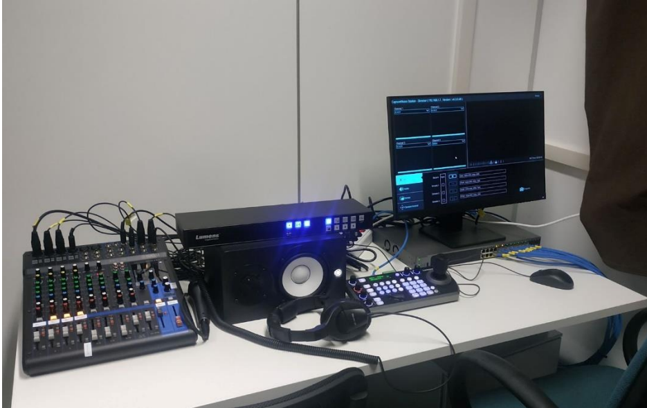
Figure 11: Electrical control unit.
